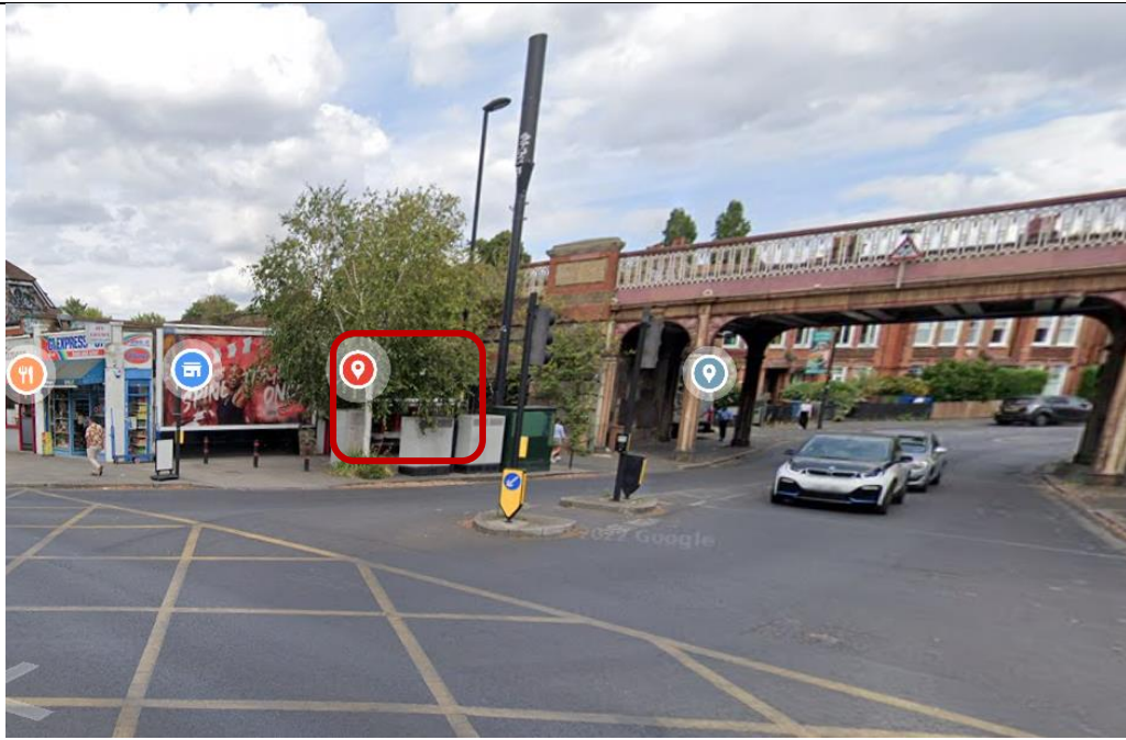
Wide shot of the corner of Croxted Road and Norwood Road, showing the communications equipment in front of number 294 Croxted Road (outlined in red).
